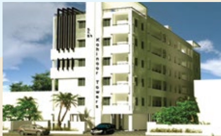
STB Kohinoor Towers, LB Nagar Hyderabad
